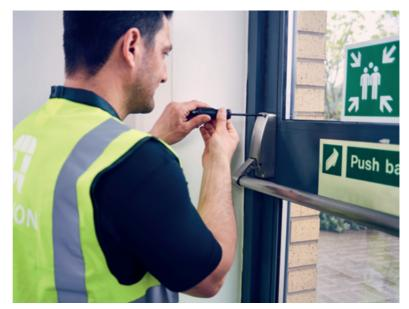
All Briton exit devices are supplied with self-tapping screws suitable for timber and metal doorsets.
